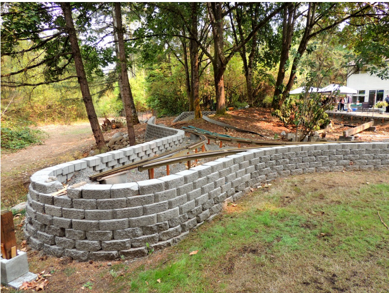
The promise of things to come - a major expansion Jerry has under construction.
