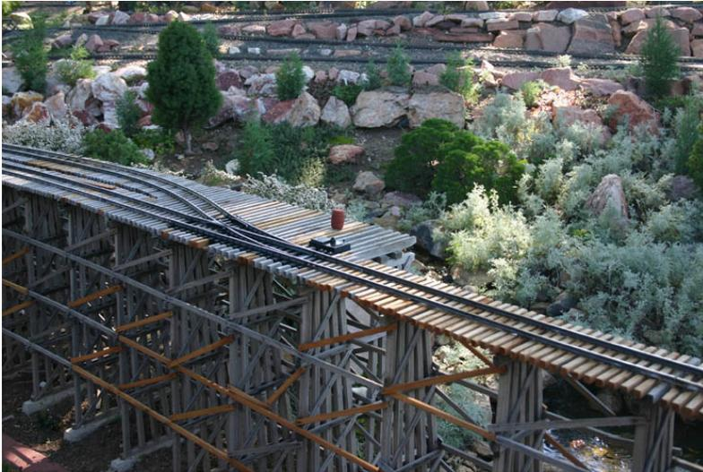
In all of the pictures, you can discern 'new' lumber from the 'old'. Structural timber has been replaced as it aged or loosened — and there's quite a bit of it. But obviously the new lumber in 2015 is not the new lumber in 2004. So what we're seeing here is a very impressive structure which the owner has taken the trouble to maintain carefully. After 11 years, it's still a crowd pleaser.
